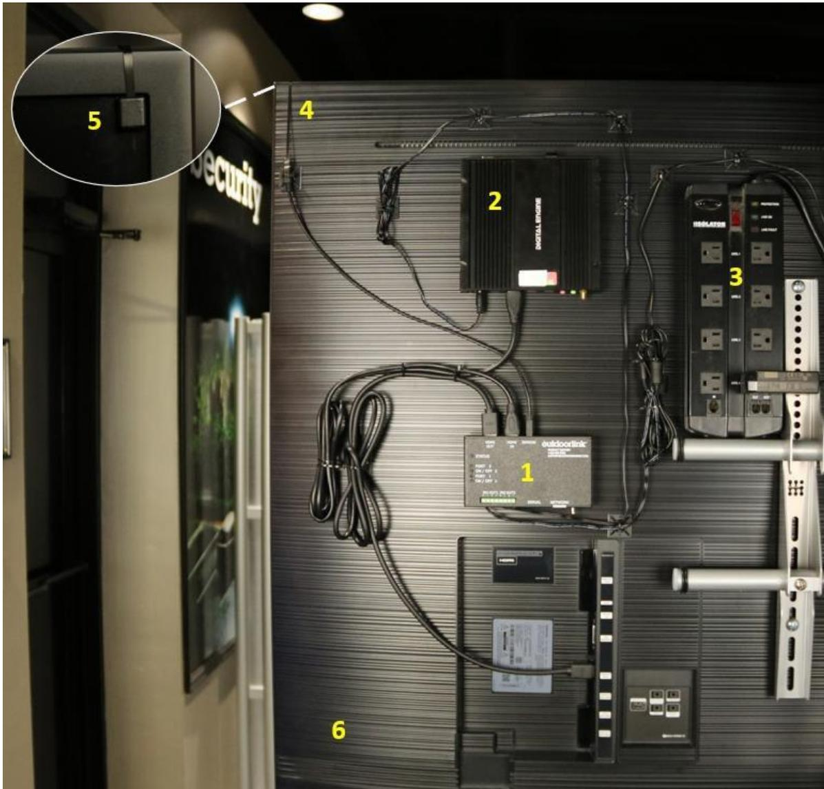
1. Vantage Controller – Positioned based on access to power, video and sensor circuits.
